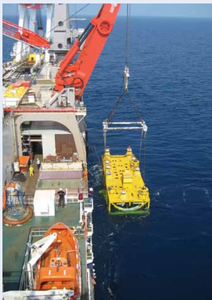
Allseas' Audacia installing a PLEM
