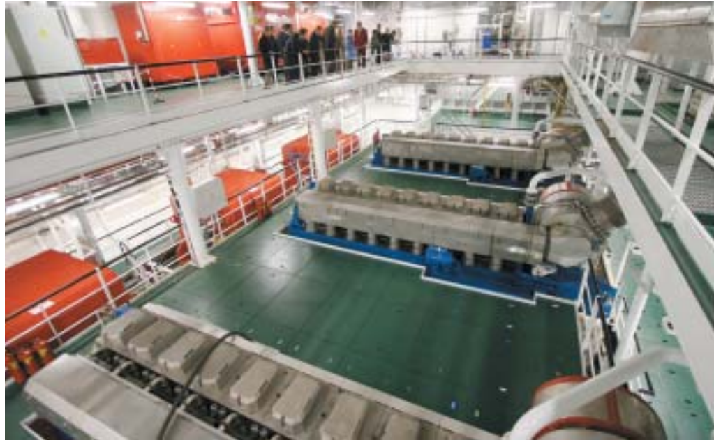
One of the two added engine rooms
